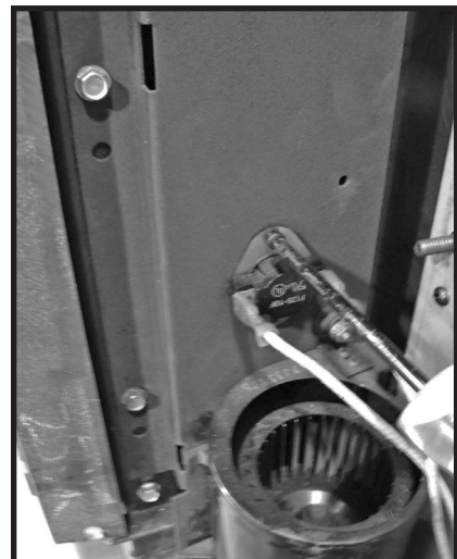
Figure 22: Unscrew thermal snap switch.
