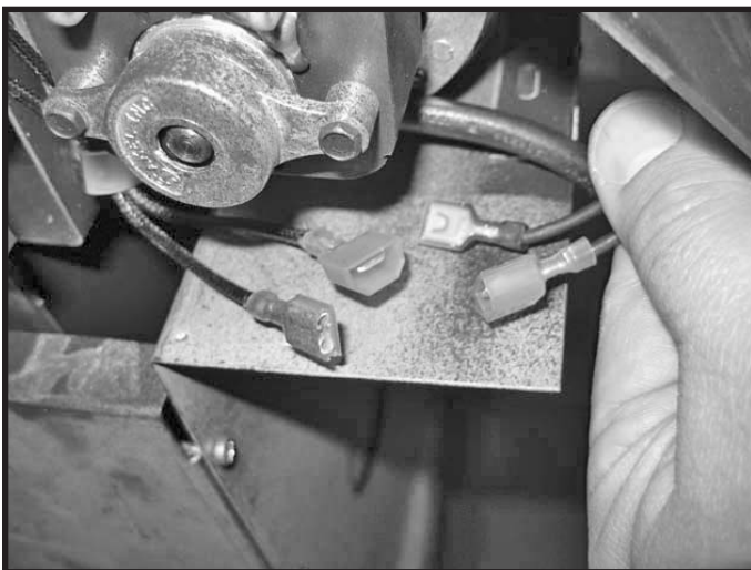
Figure 21: Disconnecting fan wires.
